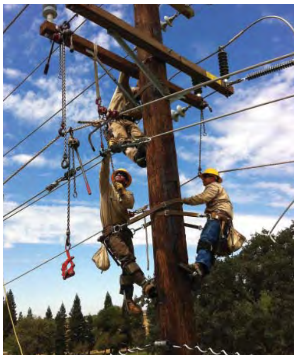
IBEW utility members working on an outside line
