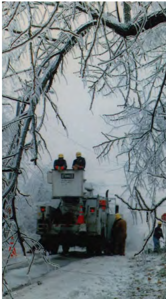
IBEW linemen and utility workers keep the power running during extreme weather
